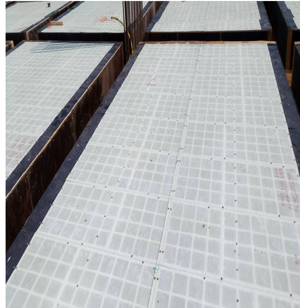
Formwork PlusDeck construction method
