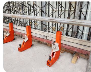
[ the bottom anchor bolt ]
